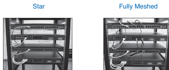
Figure 1-19 Star and Full-Meshed Topologies
